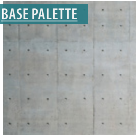
Board form concrete base
