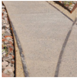
Pavers with steel edging to emulate the railroad tracks
